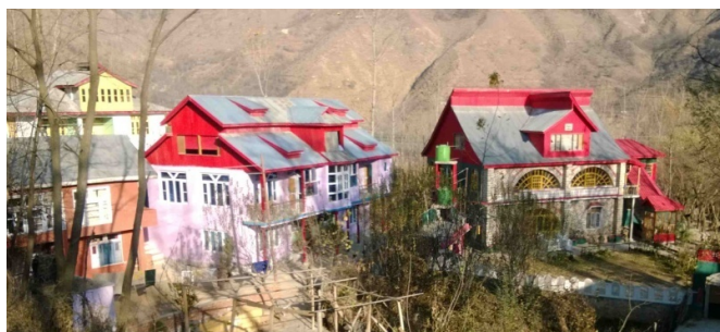
Figure 3-7: Pucca House in Planning Area
